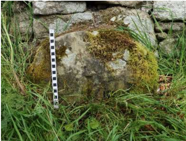
Linton, Captains Beck bridge, south side.
