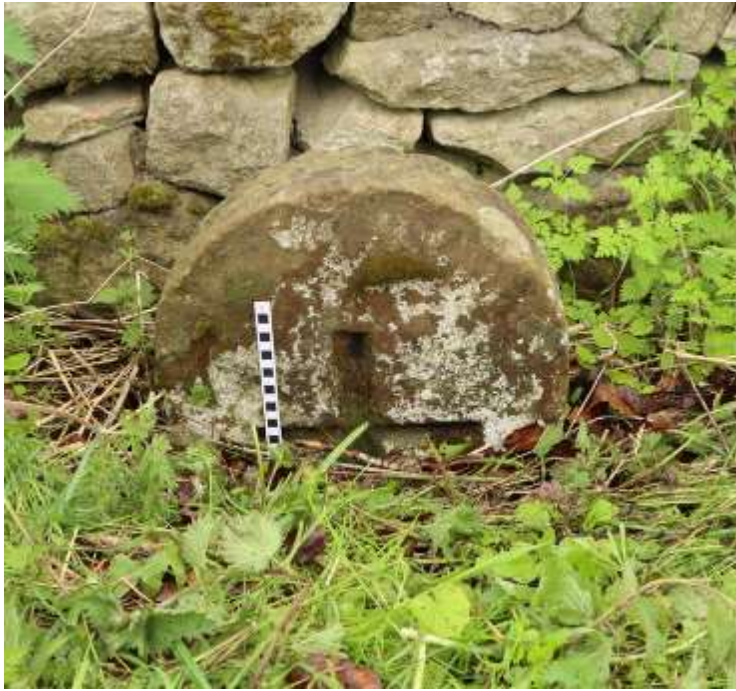
Isingdale Bridge, east side.
