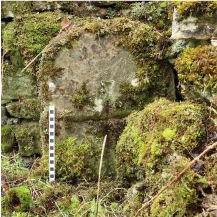
Linton, Captains Beck bridge, north side.
