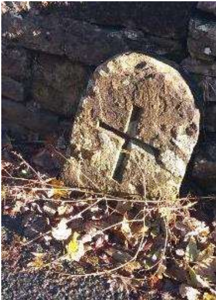
Kettlewell New Bridge, south side
