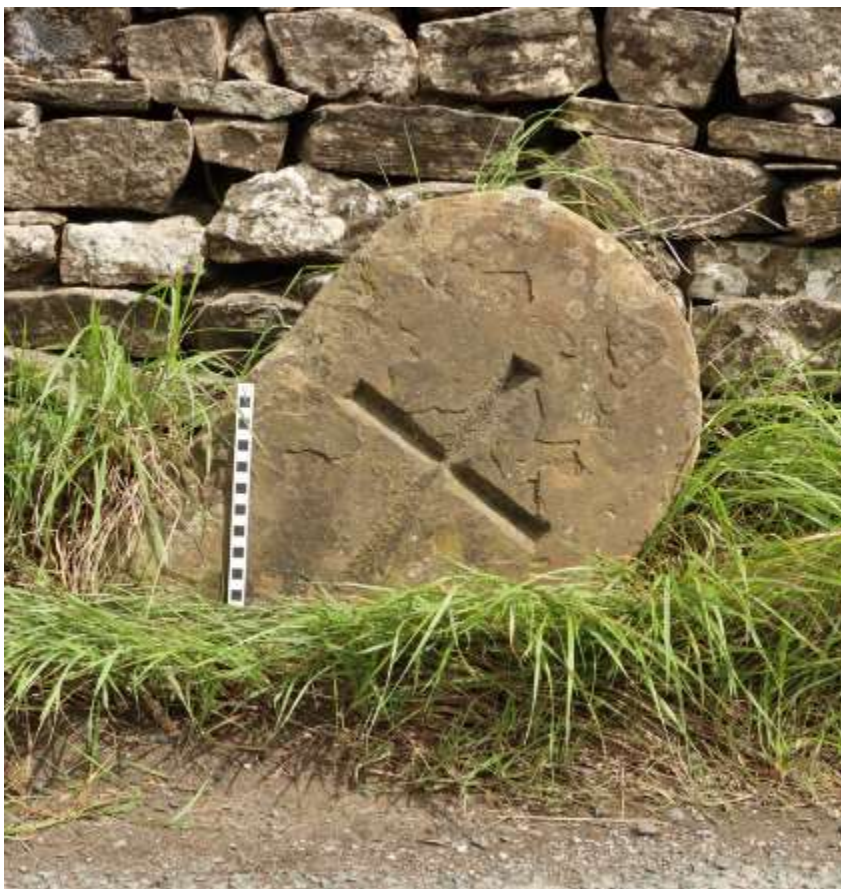
Isingdale Bridge, west side.
