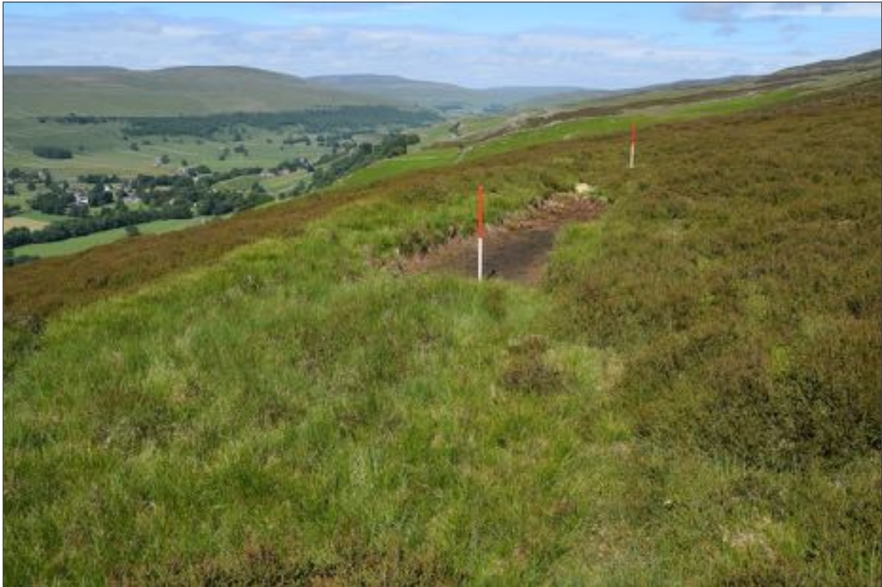
P20 - Reservoir dam. Built across the hillside (pale green vegetation). The brown area between the ranging poles is the area of the reservoir, dry when this photograph was taken. The reservoir is approximately 24m long and 3m wide and the retaining bank 0.5m high. NGR SD 94730 71791. (Scale one metre ranging poles)
