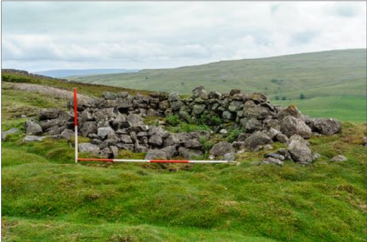
P22 - Ruined circular stone structure on the Great Spar Vein. Approximately 4m x 4m. The walls are built of sandstone blocks and are approximately half a metre thick. NGR SD 94685 71764. Looking south east. (Scale one metre ranging poles)
