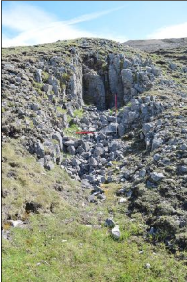
P14 - Adit (A2) - Great Spar Vein. Cut in limestone NGR SD 94542 71726. (Scale one metre ranging poles)
