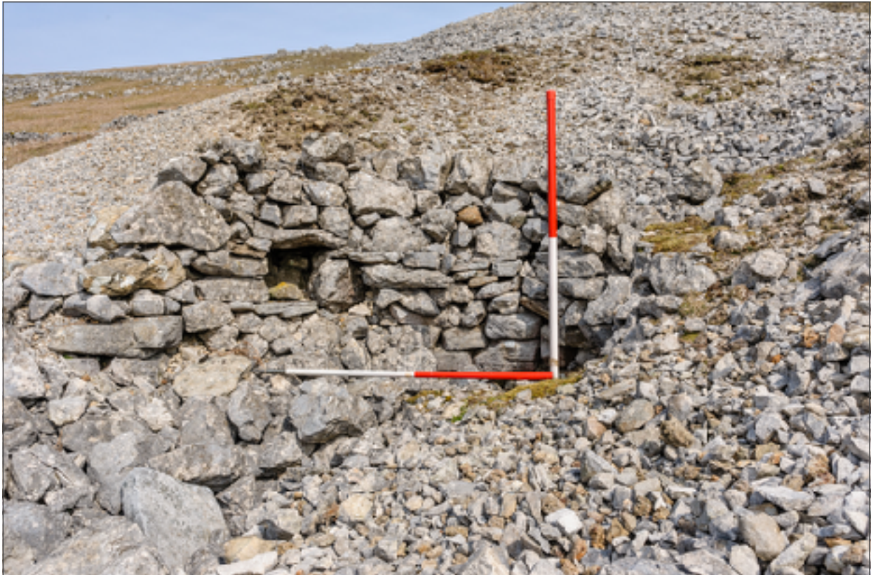
P4 - Stone structure around a filled shaft top (S1) on the Great Spar Vein. NGR SD 94581 71774. (Scale one metre ranging poles)
