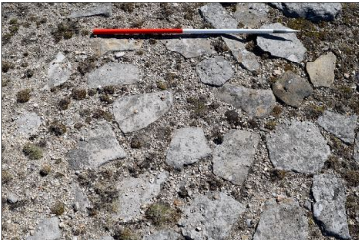
P29 - Area flagged with sandstone blocks. Dressed waste between the blocks. (Scale one metre ranging poles)
