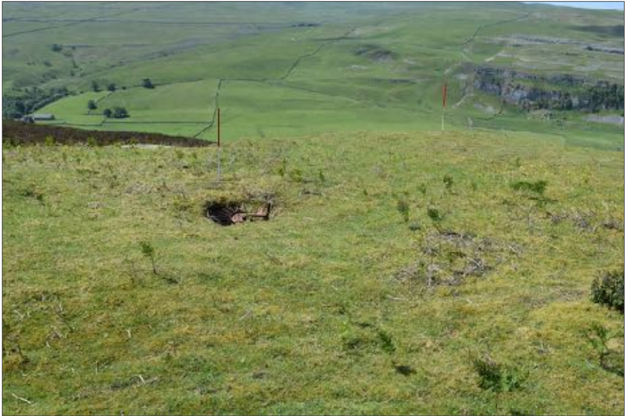
P18 - Platform at the eastern end of Blea Scar Rake with shaft. Shaft covered by a piece of old agricultural machinery (wuffler wheel from a hay tedder). The top of the shaft is stone-lined and the shaft is 8m deep. NGR SD 94888 71604. (Scale one metre ranging poles)
