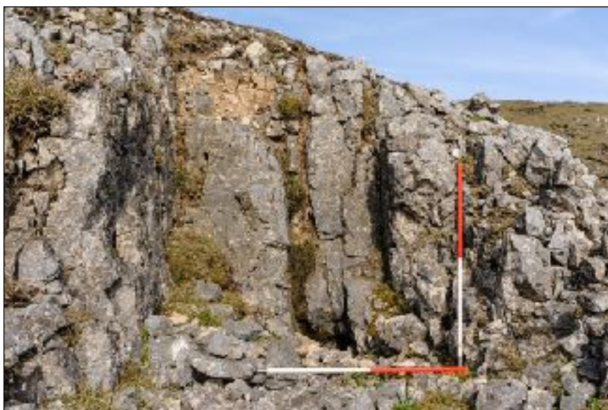
P15 - Adit (A2). Small open level behind boulders. (Scale one metre ranging poles)
