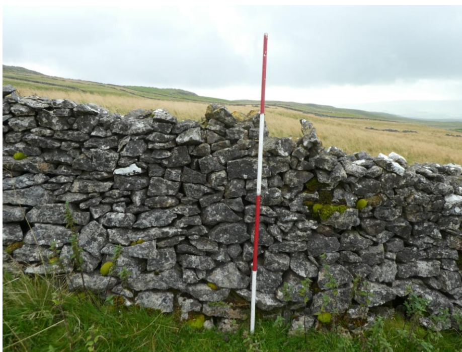
Fig. 26 Wall no. 19, a battered and low enclosure wall of 1803
