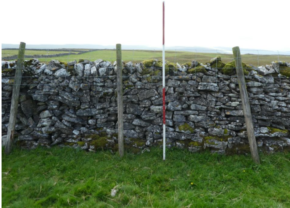
Fig. 32 Wall no. 11, a battered wall within the Enclosure area but not depicted on the 1802 map
