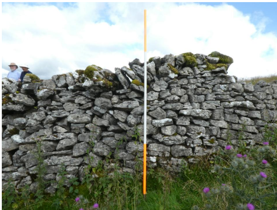
Fig. 26 Wall no. 19, a battered and low enclosure wall of 1803
