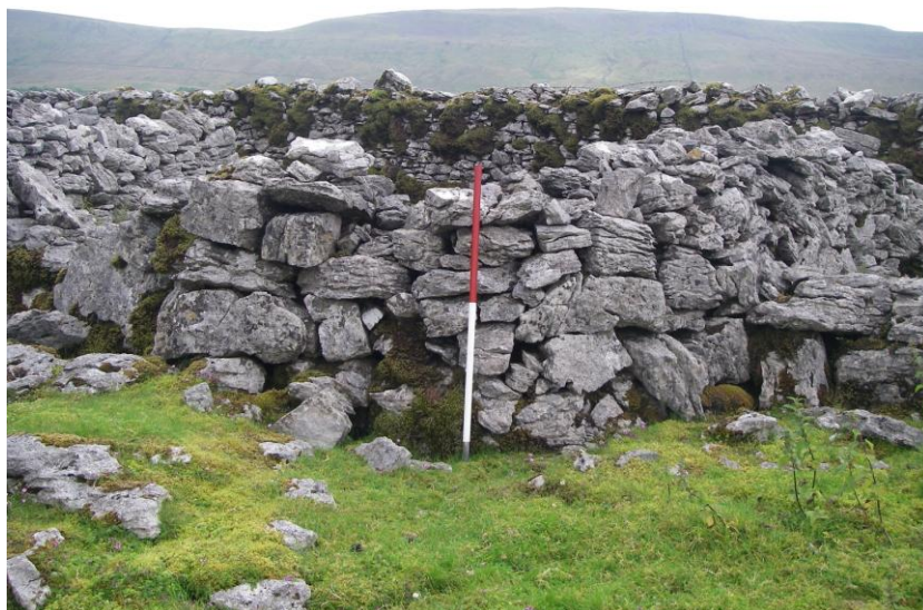
Fig. 8 A Type 1 blocky wall at Scales with later coursing at the top
