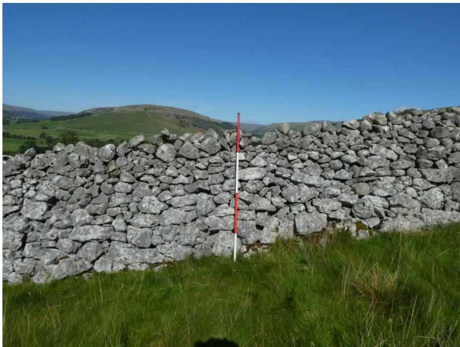
Fig. 21 Wall no. 18, a limestone-cobble wall in the former townfields
