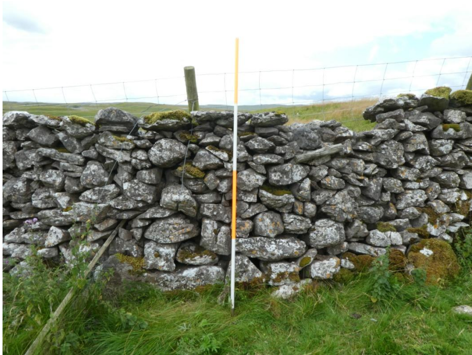
Fig. 31 Wall no. 42, an Enclosure wall built of field-clearance limestone
