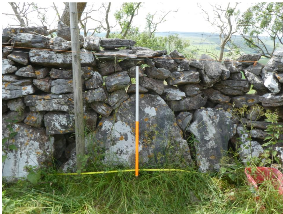
Fig. 23 Wall no. 25 in a section containing many orthostats
