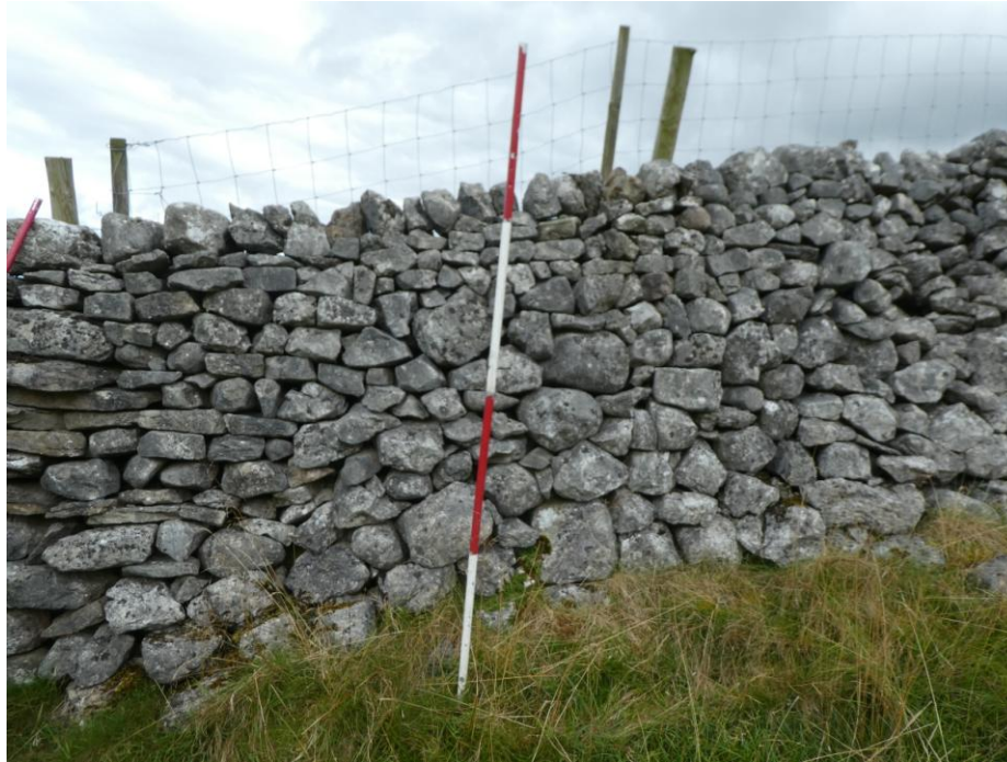
Fig. 25 Wall no. 43, a very high wall with large basal boulders
