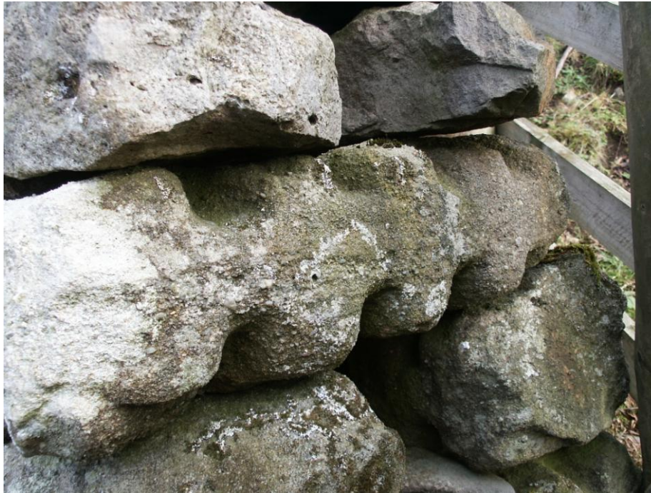
Fig. 71 Reused corn-drying kiln blocks in a wallhead on Scot Gate Lane
